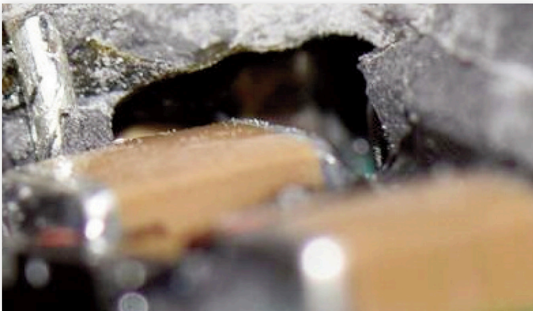
Figure 1: Example of a large air void in an encapsulated assembly
